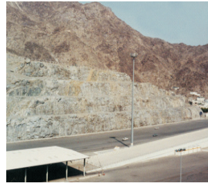
Rock Stabilization Project in Makkah
