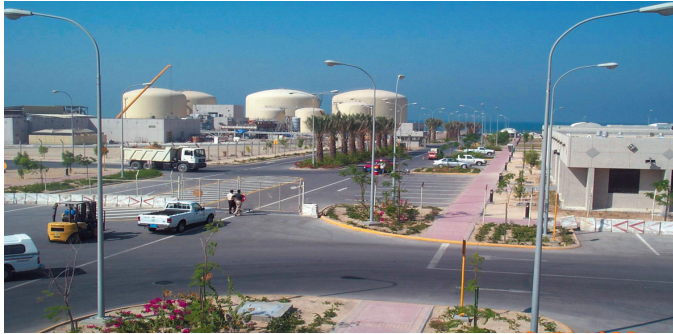
Central Administrative Service Area (CASA) At Ghazalan Power Plant.
